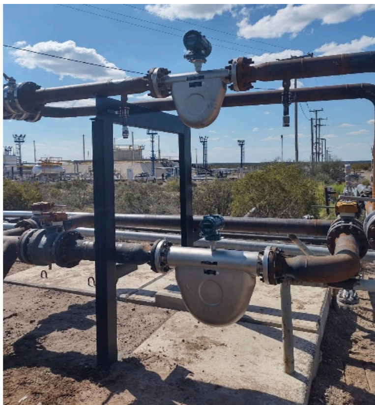
Figure 2. Rotamass meters installed.
